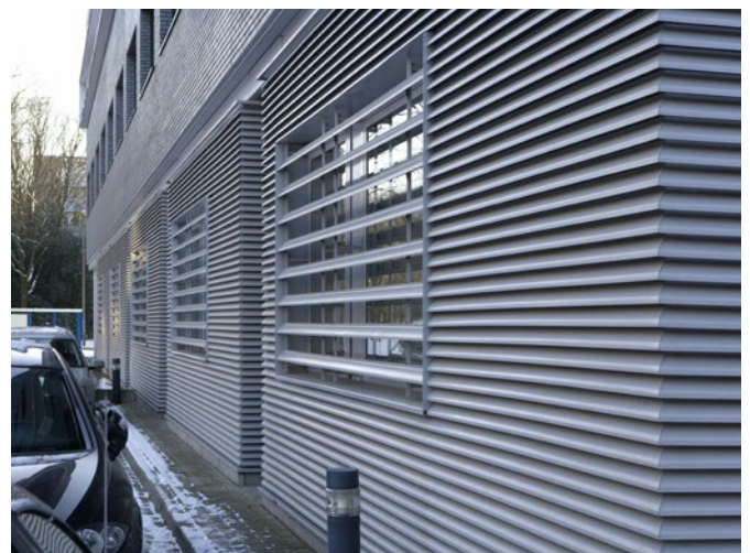
Accountantskantoor BDO, Tilburg
